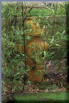
This hydrant would be hard to find in an emergency.
