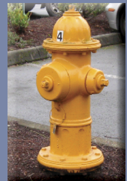
Brightly painted and cleared of debris makes this hydrant easy to find.
